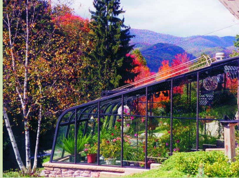
Residential horticultural greenhouse, lean-to built-up mill finish, featuring evaporative cooler, aluminum roll-up shades and gas heater.
